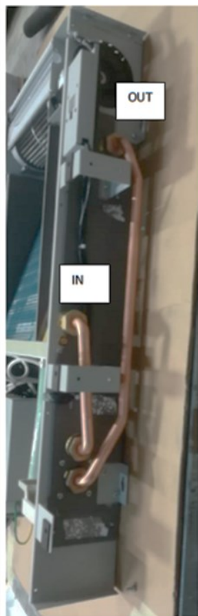
PIPE CONNECTION WITHOUT INSULATION
